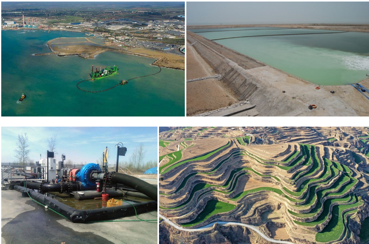
Figure 1-6. Round the clock and starting top left: Cutter Suction Dredger, large scale sediments disposal site, large scale earth works and a pumping station.
