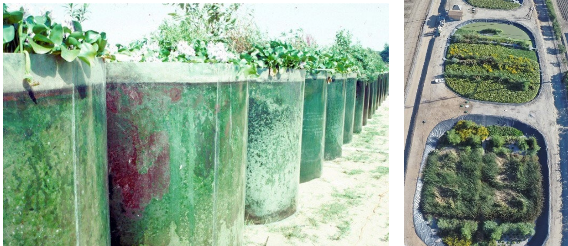
Figure 2-6. Examples of “water trains” with aquatic ecosystems (these ones are setup for waste water treatment)
